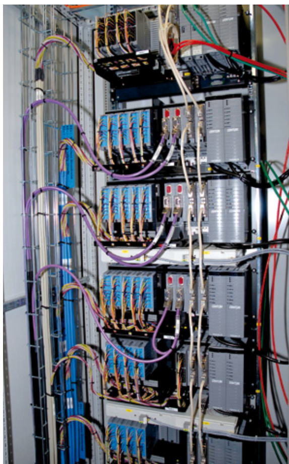
The redundant Profibus connection of the Yokogawa Centum VP control system increases availability
